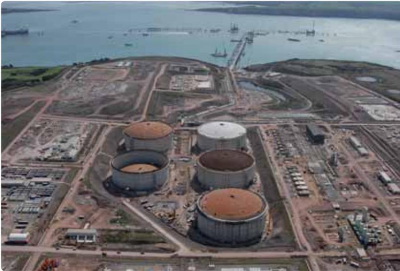
**Figure 4 above:** Liquefied natural gas (LNG) storage tanks at Milford Haven where GGBS was used at up to 65% replacement.
