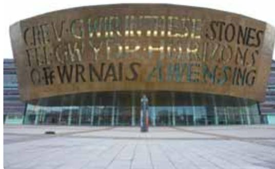
**Figure 3 left: Wales Millennium Centre, where GGBS was used at 55% replacement.**
