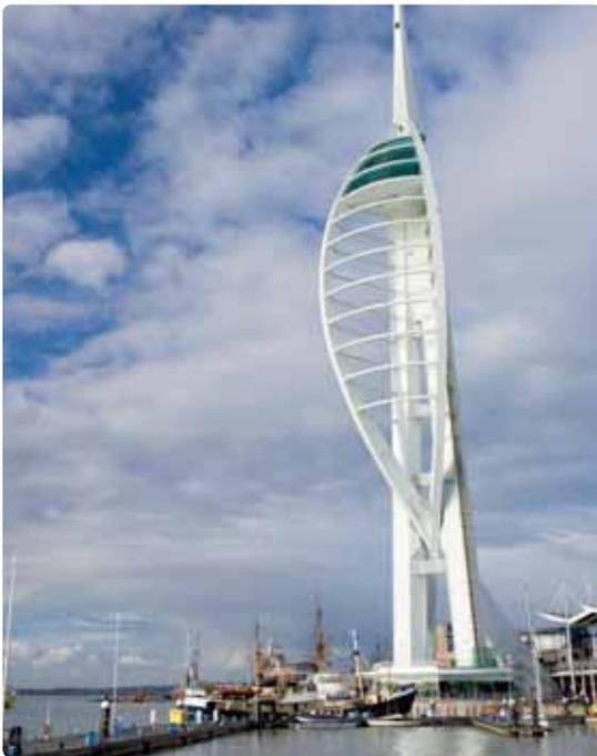
**Figure 2 far left: Spinnaker Tower in Portsmouth, where GGBS was used at 50% replacement.**
